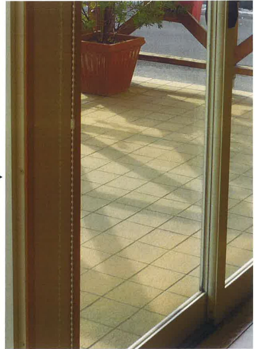
Coating is damaged by the loss of humic
